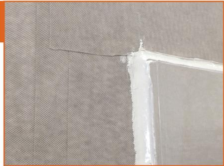
Use a compatible sealant to seal around details, reverse laps and critical areas.
