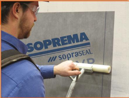
Use a roller to apply pressure over the entire surface of the membrane to ensure uniform adhesion to substrate.
