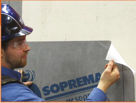
Peel off the top portion of the silicone release film and adhere the membrane to the substrate, making sure the membrane is well aligned.
